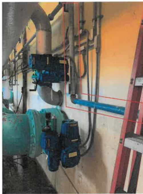
Rerouted waterline from Phase 1 at Filter 8 to accommodate air pipe penetration.
