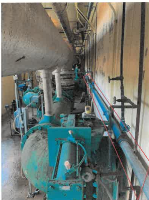
2" galvanized waterline at Filter 7 (painted blue).
