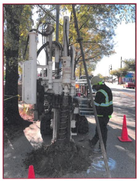
Figure 3: Mechanical Drilling and Standard Penetration Testing
