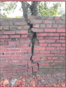
Figure 7: (L) View of Wall Along Eastern Side where Tilt is Visible. (R) Vertical Crack and Separation of Parapet Wall on Eastern Side
