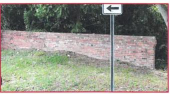
Figure 8: (L) View of Parapet Wall Along Eastern Side where Tilt is visible. (R) View of Curved Parapet Wall Along Western Side North End.
