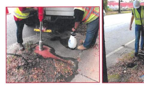
Figure 2: (L) Concrete Coring. (R) Hand Auger & Dynamic Cone Penetrometer Testing
