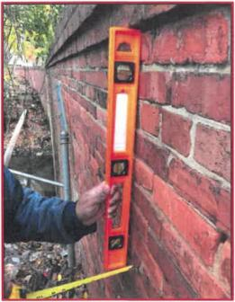
Figure 5: (L) View of Wing and Spandrel Walls along Western Side. (R) Measuring Degree of Tilt
